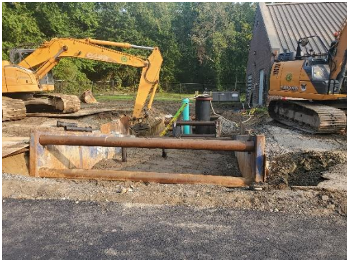
Photo 3: Trench Backfilling at the Auburn Street Pump Station
