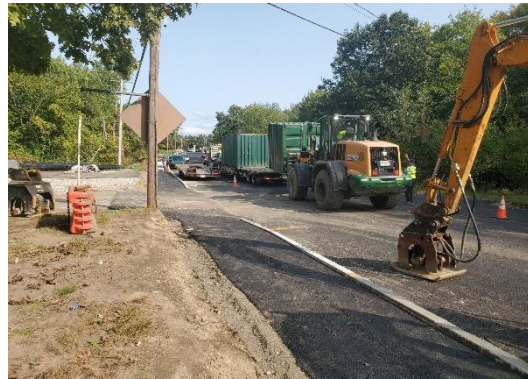
Photo 4: Material Compaction at the Auburn Street Pump Station
