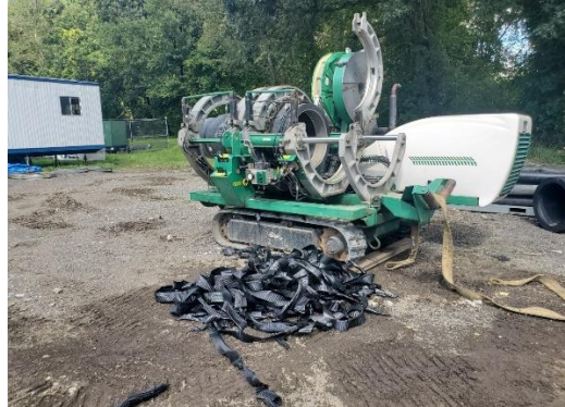
Photo 2: Setting up Varitech's HDPE Fusing Equipment
