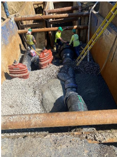
Photo 3: Installation of Launching Barrel
