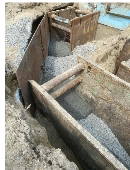
Photo 4: Trench Backfilling at Auburn Street Pump Station
