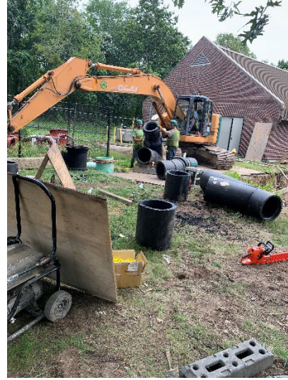
Photo 2: Assembly of 20-Inch HDPE Force Main
