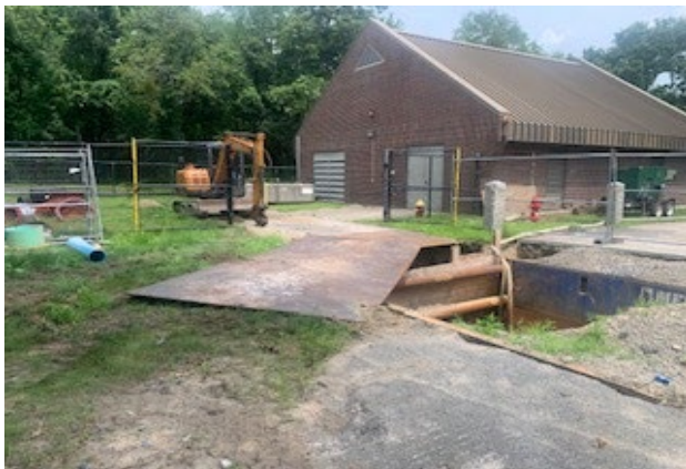
Photo 3: Excavation Activities for Auburn Street Pump Station Tie-In Connection
