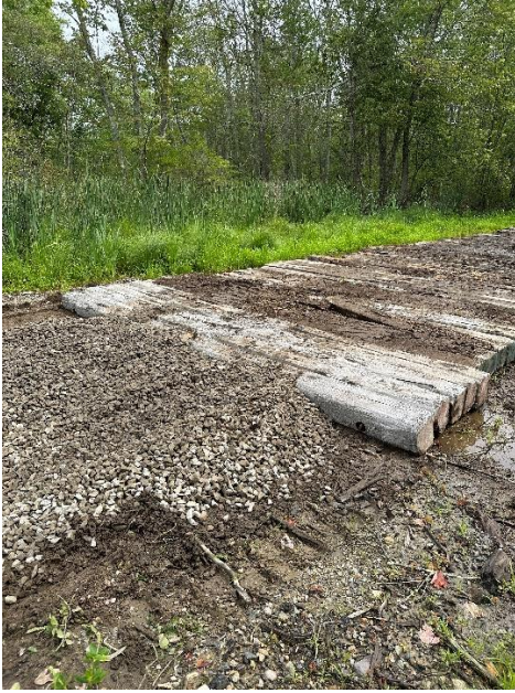
Photo 1: Timber Mats installation at Easement Near Alger Street
