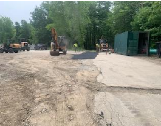
Photo 3: Pavement Restoration at C. Naughton's Staging Area
