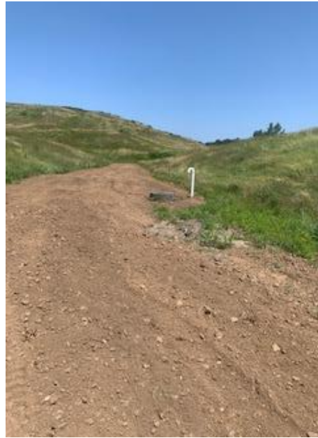
Photo 2: Landfill Restoration Near Southfield Drive
