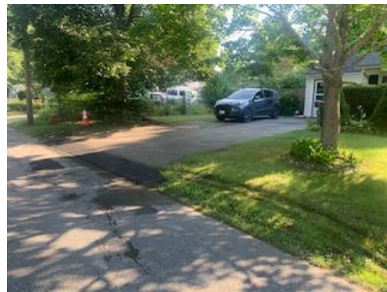
Photo 4: Driveway Restoration on Homeland Drive
