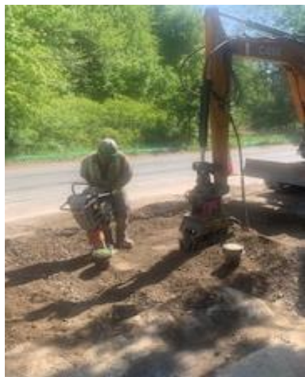
Photo 4: Trench Backfilling and Material Compaction at Auburn Street Pump Station
