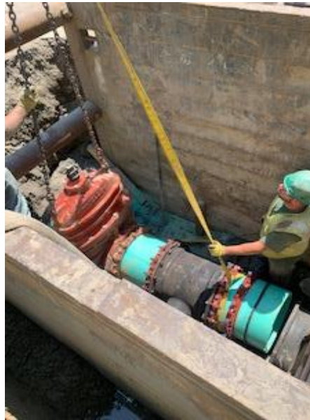
Photo 2: Installation of 20"x8" Tee and 8" Gate Valve
