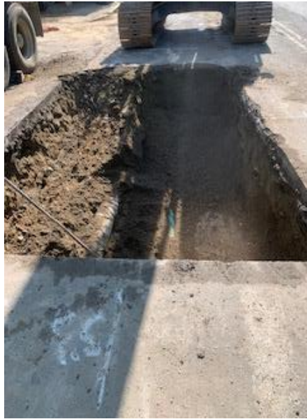
Photo 1: Excavation at Auburn Street Pump Station
