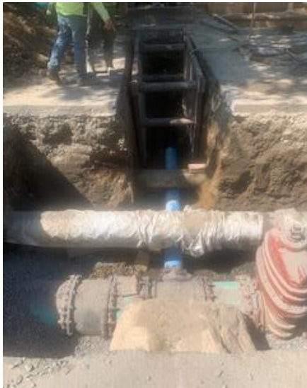
Photo 3: Installation of 8" Gate Valve and Pipe for Bypass Connection
