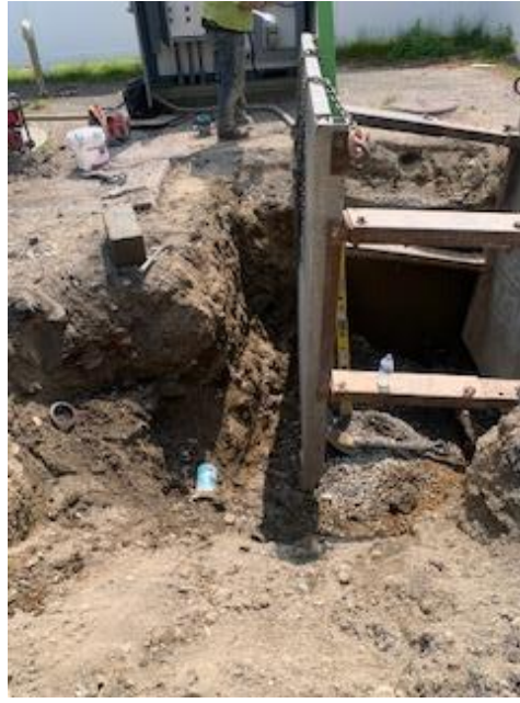
Photo 2: Excavation to Expose Pipes at Auburn Street East PS
