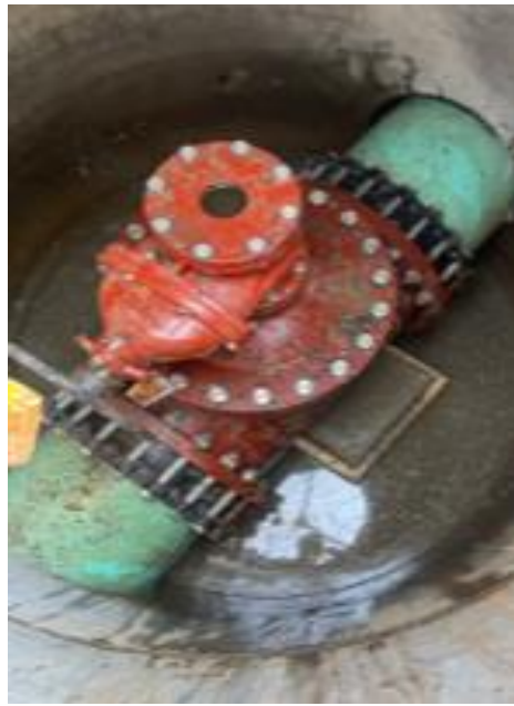
Photo 4: Concrete Cradle Installation
