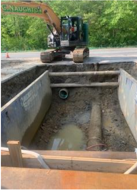
Photo 1: Excavation to Expose Existing Force Main at Auburn Street PS
