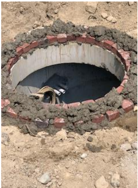
Photo 3: Flow Meter Conduits and Cables Installation
