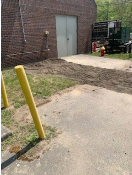
Photo 1: Trench Backfilling at Auburn Street Pump Station
