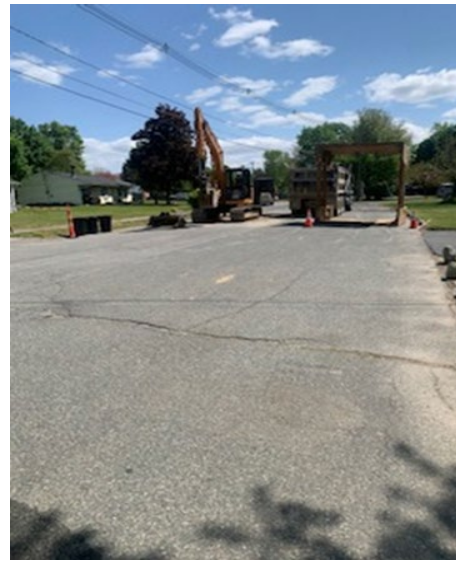
Photo 4: Mobilization of Equipment on Southfield Drive
