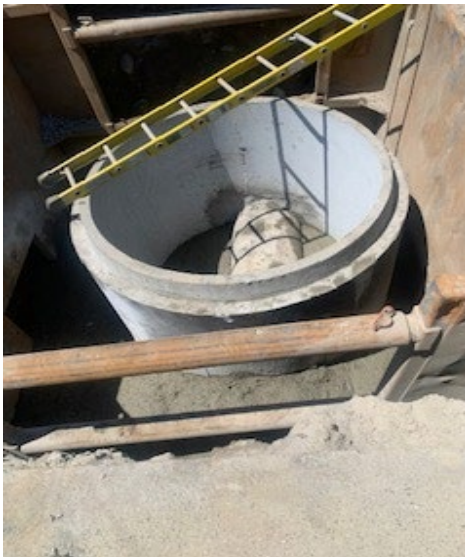
Photo 3: New Sewer Manhole with Concrete Collar on Southfield Drive
