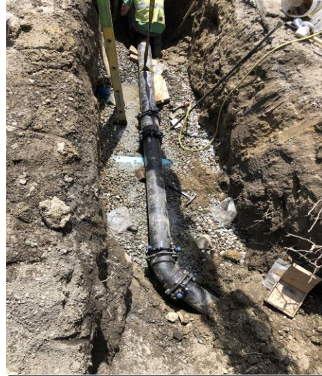
Photo 2: 6" DI Water Service Connection at 1245 Auburn Street
