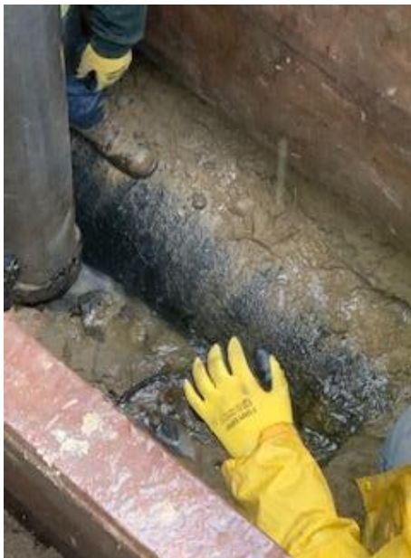
Photo 3: Existing DI Force Main Near Auburn Street Pump Station
