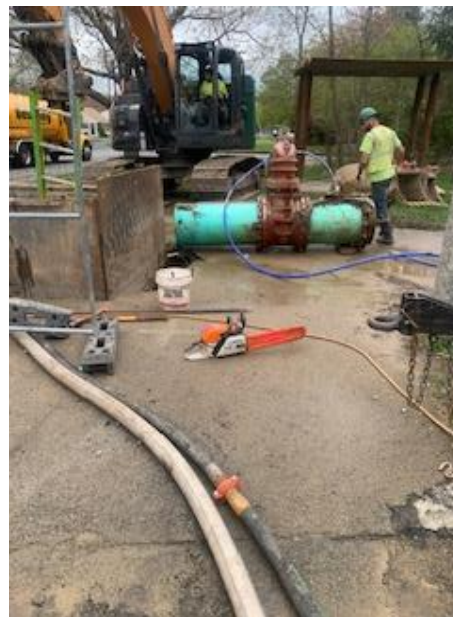
Photo 4: Replacement of New Force Main End Pipe and Gate Valve
