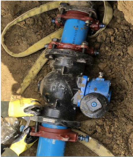
Photo 1: Installation of 4" Plug Valve near Auburnville Way
