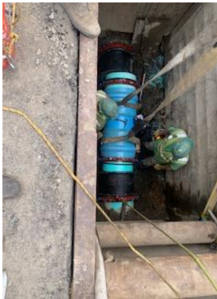
Photo 3: Installation of Tee at Captain Allen Way
