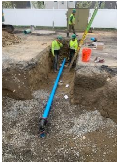
Photo 4: Installation of 4" PVC Pipe at Captain Allen Way
