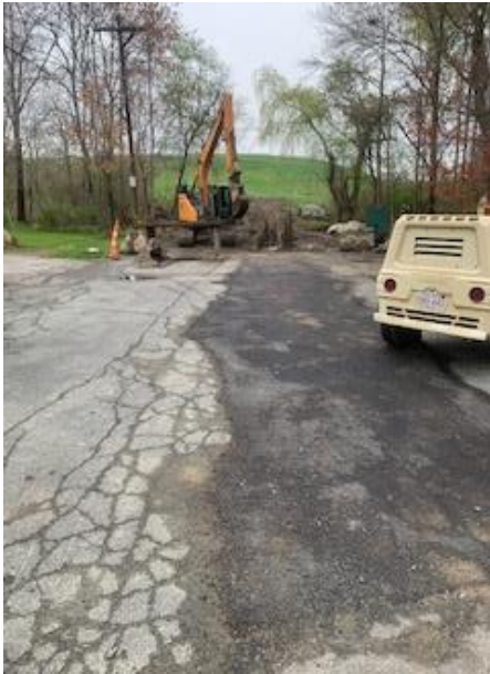
Photo 1: Cleanup at Southfield Drive
