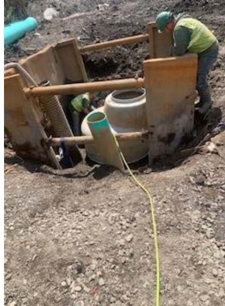
Photo 2: Installation of Epoxy Cone at Cleanout Manhole
