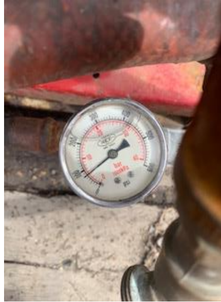
Photo 2: 20" HDPE Sewer Force Main Pressure Testing
