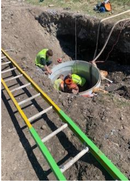
Photo 1: Gasket Leak Repair
