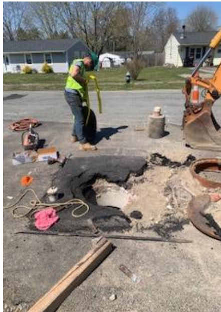
Photo 3: Sewer Force Main End Cap Installation
