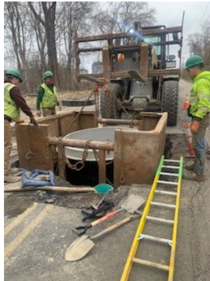
Photo 4: Installation of Manhole Riser
