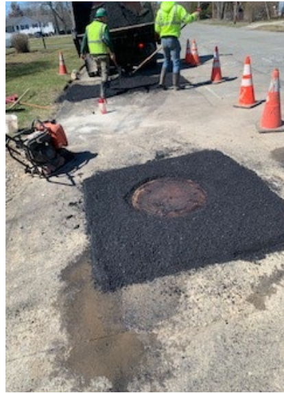
Photo 2: Installation of Manhole Rim and Cover
