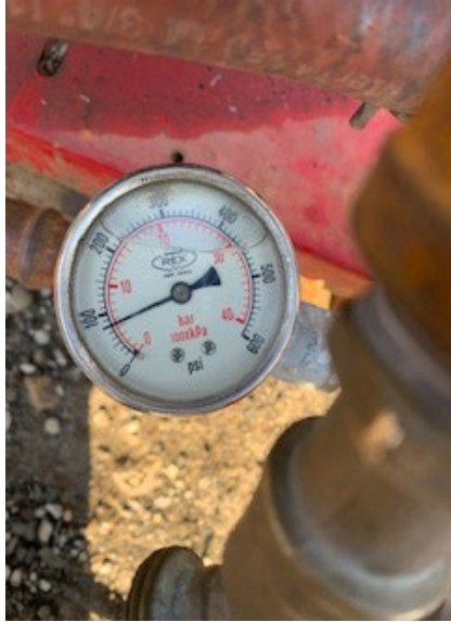
Photo 1: Force Main Pressure Testing
