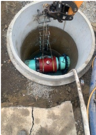
Photo 3: Installation of Fittings Inside Blowoff/Cleanout
