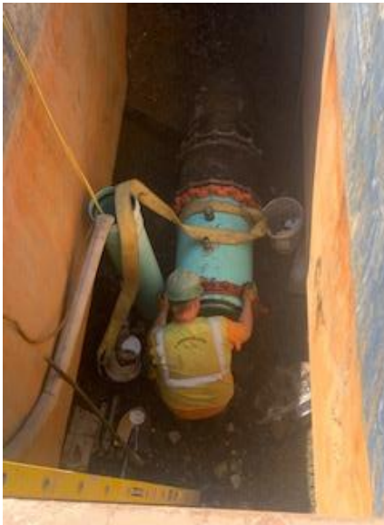
Photo 3: Installation of 2" HDPE Water Pipe Connection
