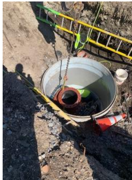
Photo 4: Installation of 20"x20" Tee Inside Air-Release Manhole
