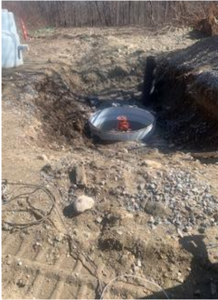
Photo 1: Installation of 6" Gate Valve Inside Air-Release Manhole
