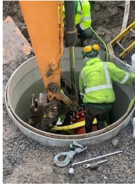
Photo 2: Installation of 20"x8" Tee Inside Blow-off Cleanout Manhole
