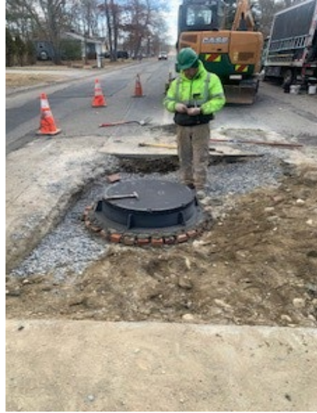
Photo 2: Installation of Air-Release Manhole Frame and Cover
