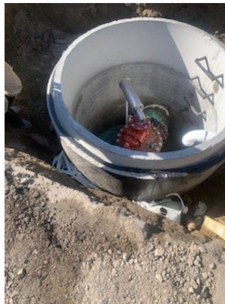
Photo 4: Installation of Air Release Valve Inside Manhole
