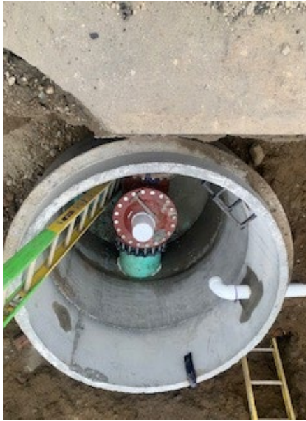
Photo 1: Installation of Air-Release Fittings inside Air-Release Manhole
