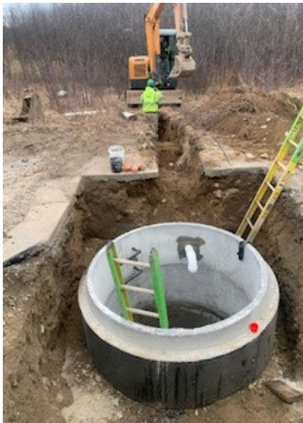
Photo 3: Installation of 4" PVC Manhole Air Vent
