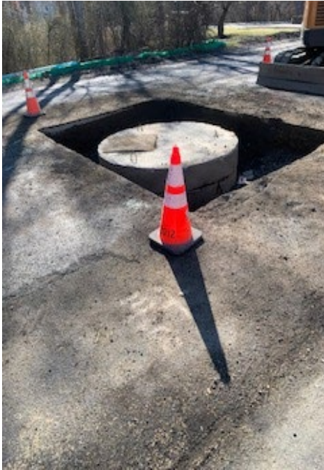
Photo 1: New Top Slab at Air Release Manhole
