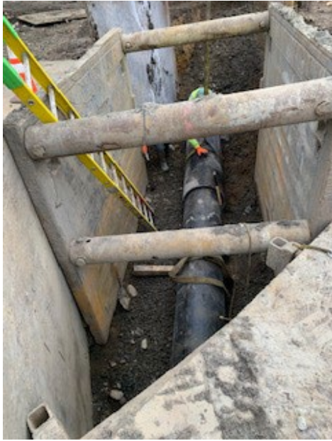
Photo 1: DI Sleeve for HDPE Force Main at 36-Inch Water Main Crossing
