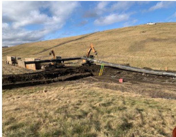
Photo 3: Fusing of HDPE Pipe in Landfill Easement
