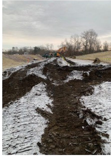
Photo 2: Trench Backfill Restoration in Landfill Easement
