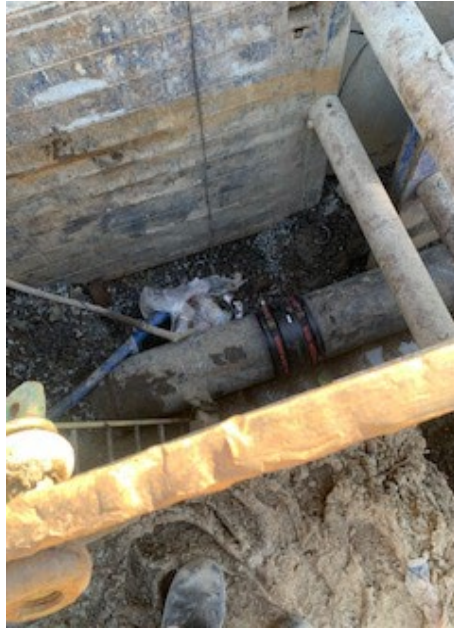
Photo 1: HDPE Electrofusion Coupling Installation
