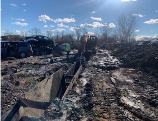
Photo 2: Trench Excavation in Junk Yard Easement
