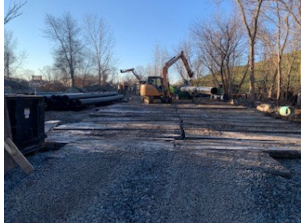
Photo 3: Timber Matting set up in Junk Yard Easement
