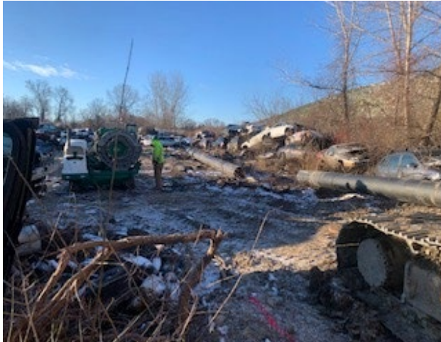
Photo 2: Crew Setting Up Fusing Machine in Junk Yard Easement
