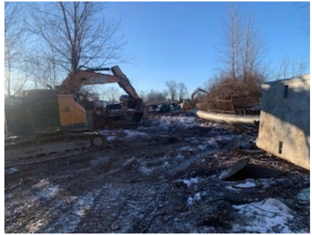
Photo 3: Trench Excavation in Junk Yard Easement
