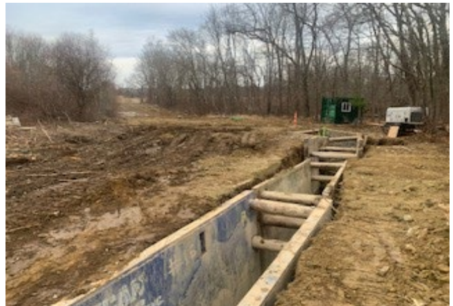
Photo 3: Force Main Excavation Support
