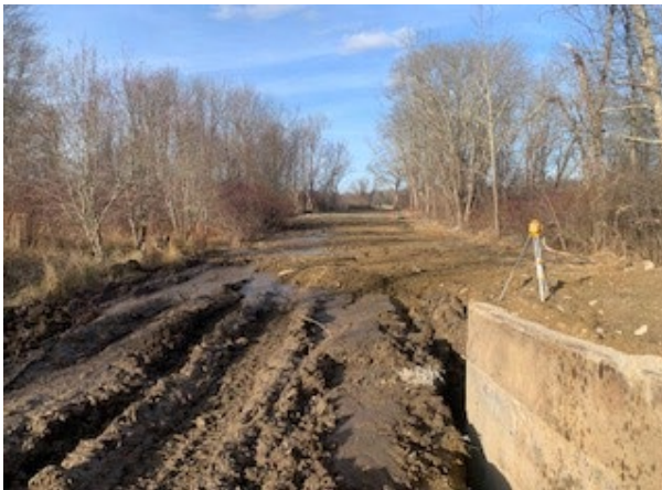
Photo 2: Easement Grading and Restoration
