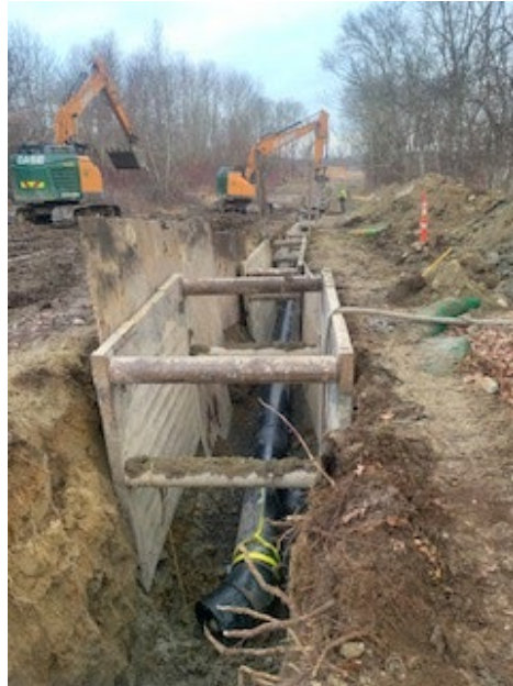
Photo 1: Sewer Force Main Installation in Thatcher Street Cross-Country Easement
