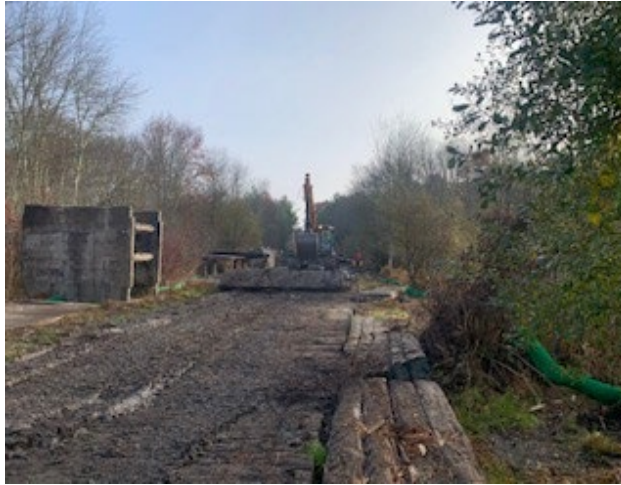
Photo 1: Timber Matting Removed to Allow for Force Main Installation
