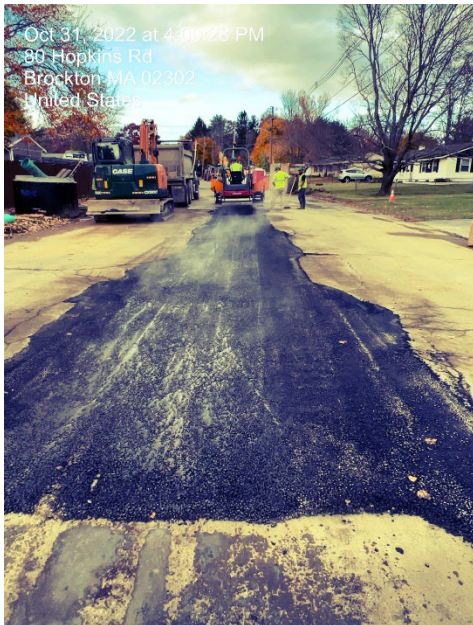
Photo 2: Paving of Sewer Trench on Southfield Drive
