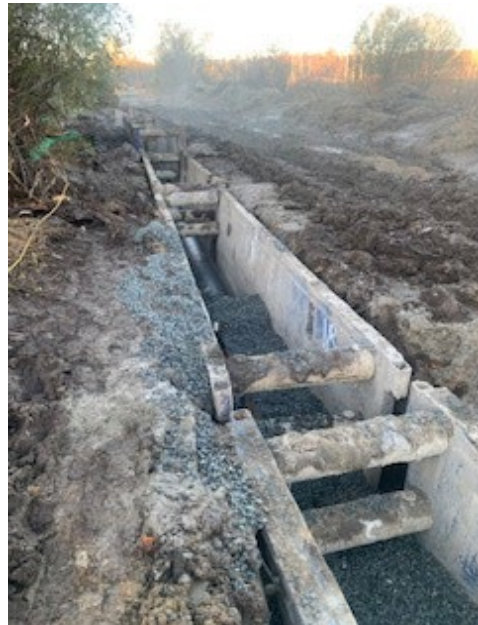
Photo 3: Excavation Support for Sewer Force Main in Cross-Country Easement
