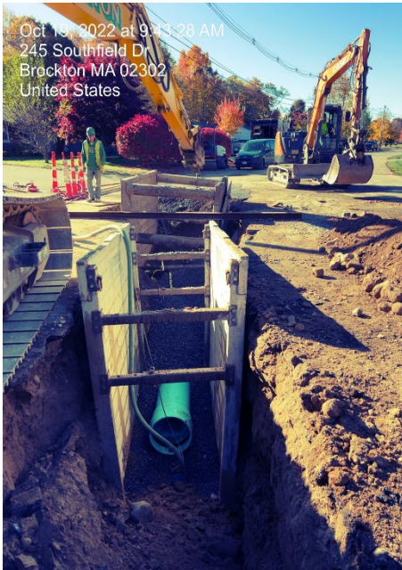
Photo 2: New Sewer Force Main Installation on Southfield Drive
