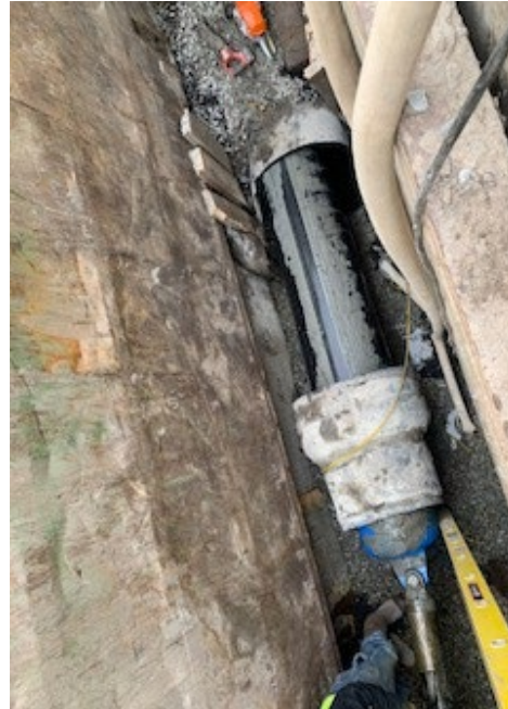
Photo 3: 20" HDPE Force Main Successfully Pulled across Beaver Brook
