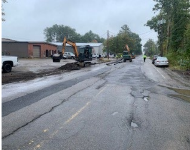
Photo 1: Removal of Water Main Bypass Piping on Auburn Street
