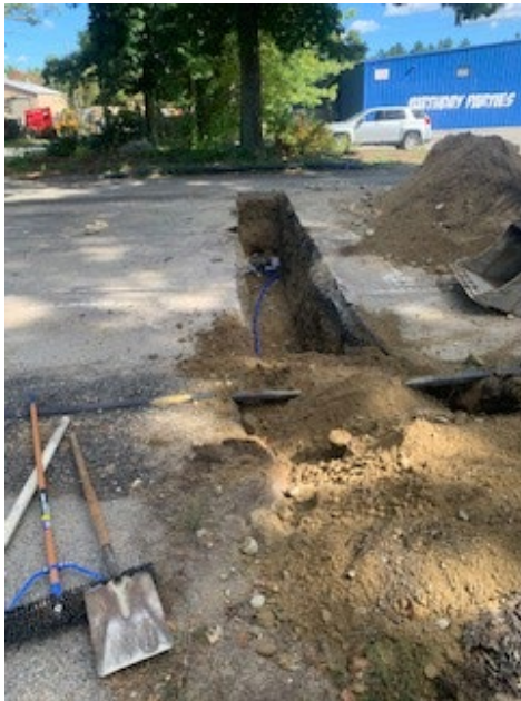
Photo 2: Water Service Installation Work on Auburn Street
