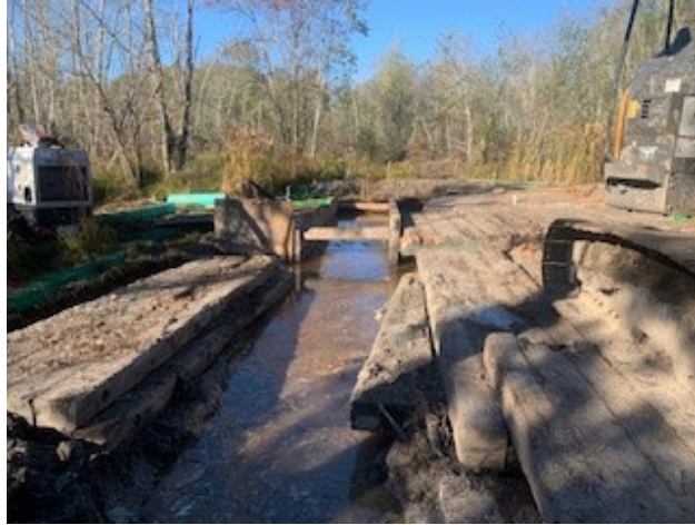
Photo 1: Receiving Pit for Directional Drilling Work in Cross-Country Easement
