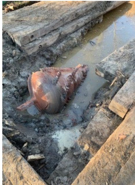
Photo 3: 36" Reamer for Directional Drilling work in Cross-Country Easement
