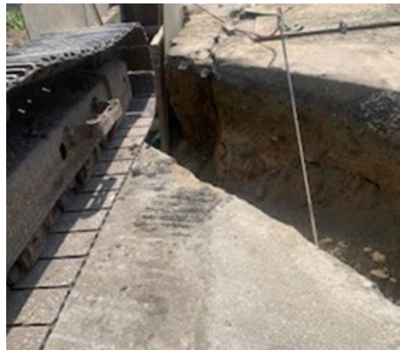
Photo 3: Trench Excavation at 45 Degree Bend
