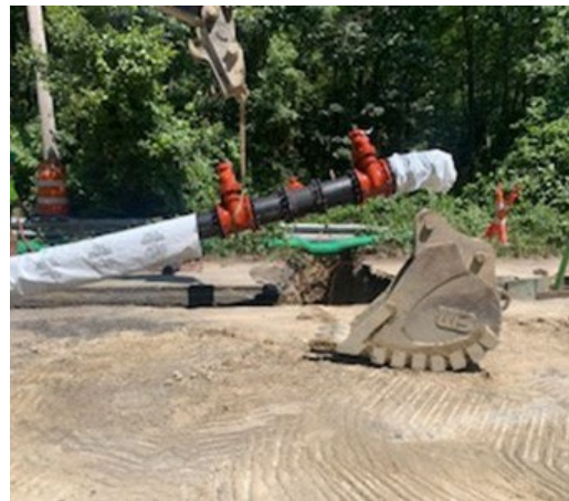
Photo 3: Installation Valve Assembly on Auburn Street
