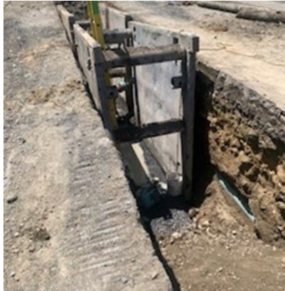
Photo 1: Installation of 12-inch DI Water Main on Auburn Street
