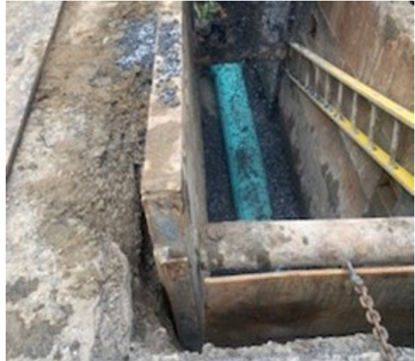
Photo 3: Installation of 20-inch PVC Sewer Main on Auburn Street
