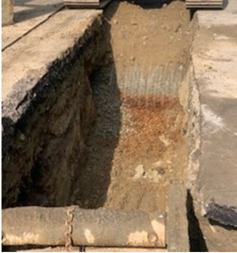
Photo 2: Excavation of Culvert at STA 19+50 during 20-inch PVC Sewer Pipe Installation
