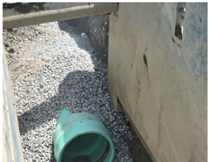
Photo 2: Crushed Stone Placed After Pipe Installation
