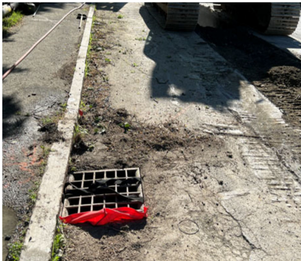
Photo 1: Silt Sack Erosion Control Installation
