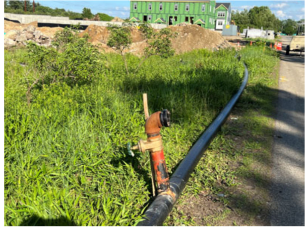
Photo 4: 6" Temporary Bypass Piping Connected to Temporary Hydrant
