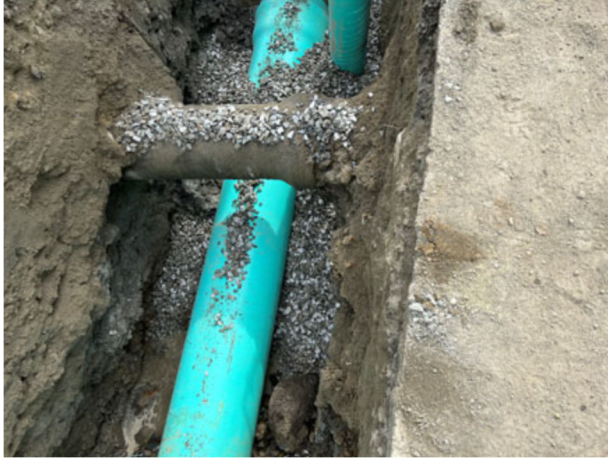
Photo 3: Newly Installed 20" PVC Sewer Main Under Drain Crossing
