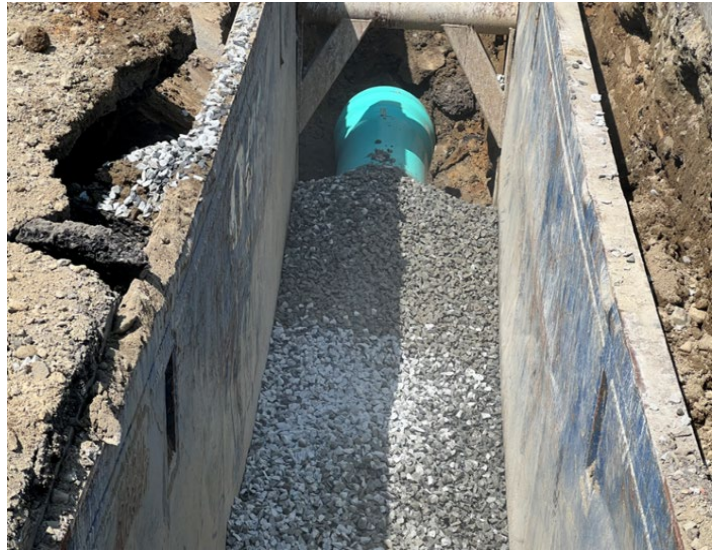
Photo 2: Crushed Stone Placed After Pipe Installation
