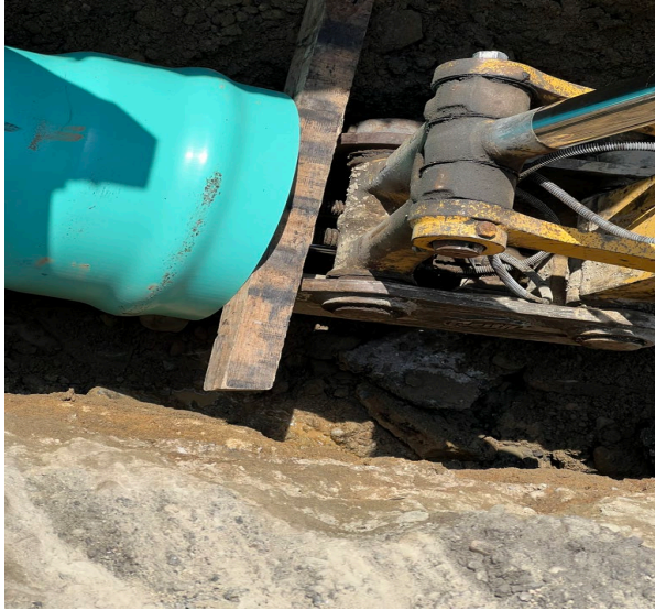
Photo 1: 4X4 Protecting Pipe from Damage during Installation
